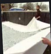
Fitting of the liner
